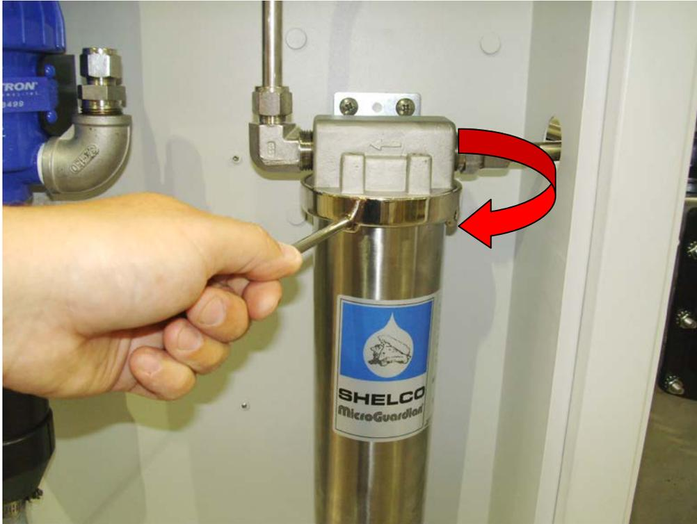
Remove the filter housing and collar.
