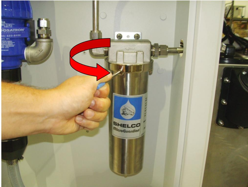
At this point the filter replacement is complete, and the machine can be turned back on. It is a good idea to reset the maintenance reminder on your startup screen. This is done by pressing the drain filter button on the display.
