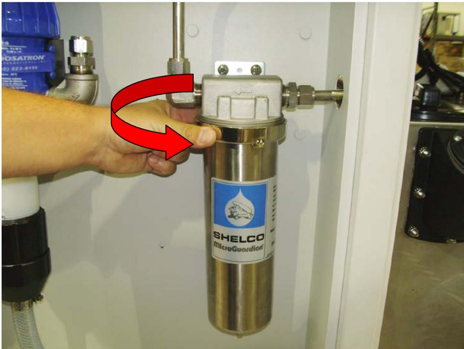
Tighten collar using the tool provided.
