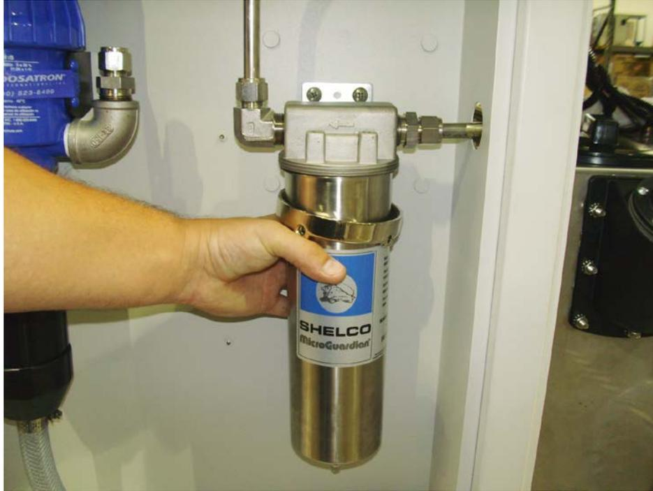
Screw the collar back onto the filter head to the right by hand.
